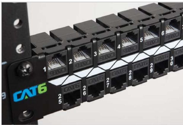
The top and bottom rows have couplers oriented in opposite directions
