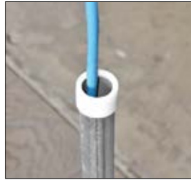
SNAP ON BEFORE CABLE PULL
