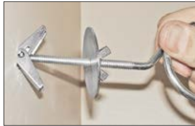
TOGGLE IN...TIGHTEN DOWN
