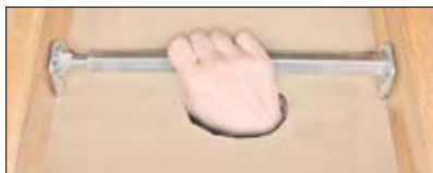
2) TWIST OUT TO BITE ON JOISTS
