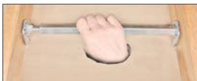
2) TWIST OUT TO BITE ON JOISTS
