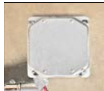
PROTECTED READY FOR DRYWALL
