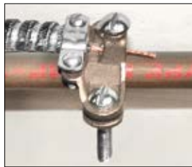
CLAMP SECURES BX/MC IN PLACE
