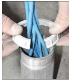
FOR THREADED CONDUIT/CONNECTORS
