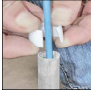
SNAP ON BEFORE OR AFTER CABLE PULL
