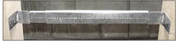
TELESCOPING SCREW GUN BRACKET IN WALL OPENING
