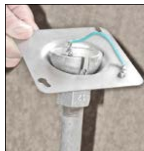
BOND WIRE CONNECTS COVER AND PIVOT BALL
